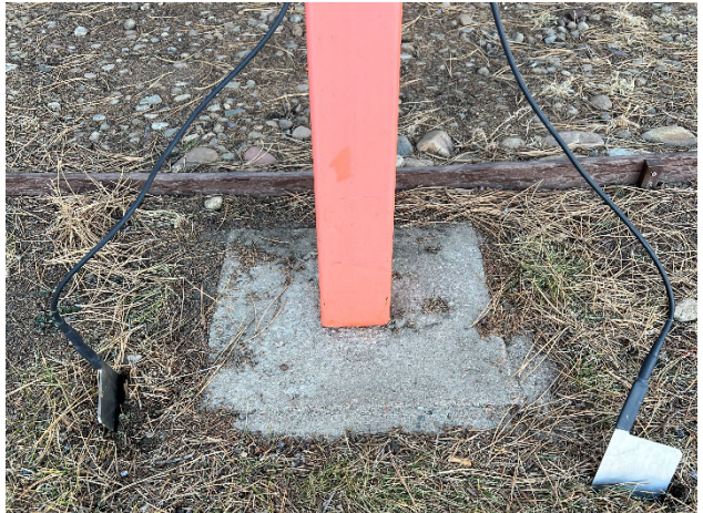
Figure 2-2: Mud Plugs in Use
